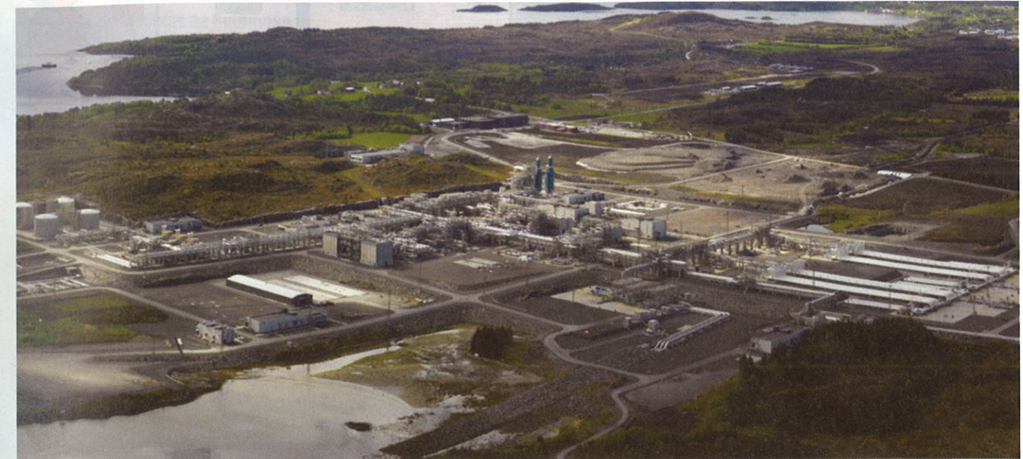
The Ormen Lange Plant on Nyhamna Island, Norway.
